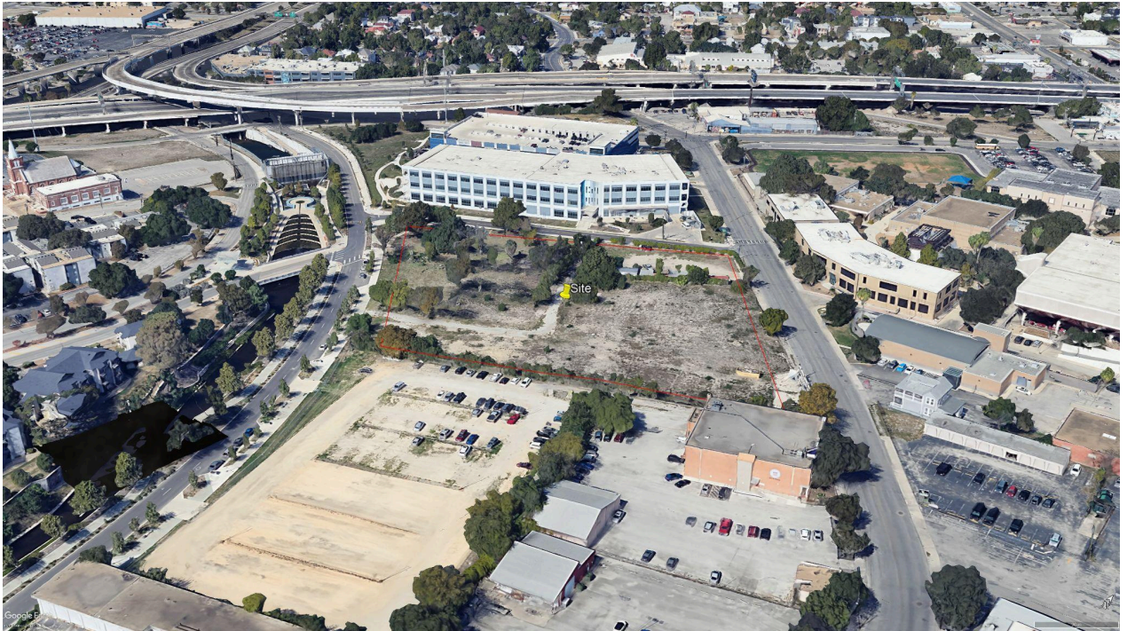
Figure 2.1.6.1. View from southeast (Google Maps, 2025)
