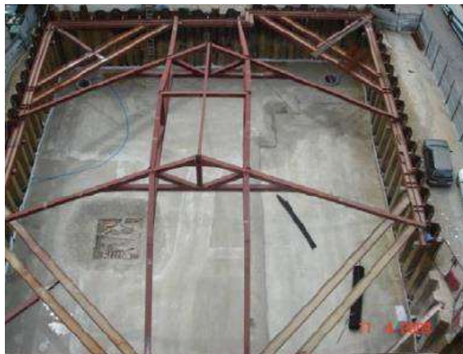
Figure 3.28. Braced steel sheet piles example (Athanasopoulos, 2011).
