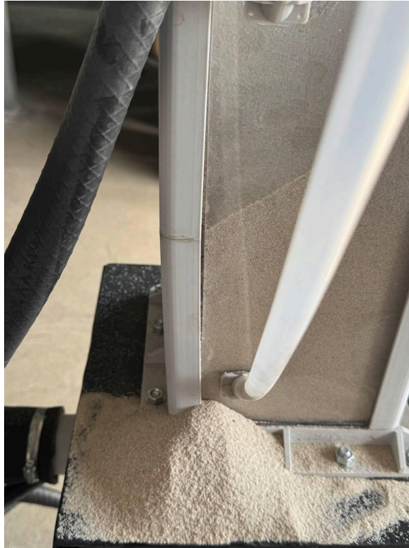
Figure 42. Structural failure on the FR.
