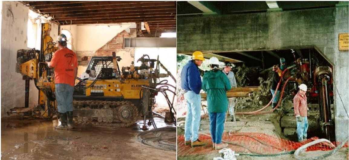
Figure 4.28. Installation of micropiles by drilling machine.
