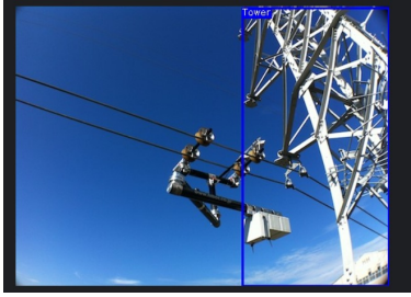
(a) Pre-trained baseline: tower class detected at high confidence on a real inspection photograph showing conductors and tower hardware.
