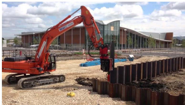
Figure 4.12.2 Sheet pile driving using hydraulic hammer (from google website)
