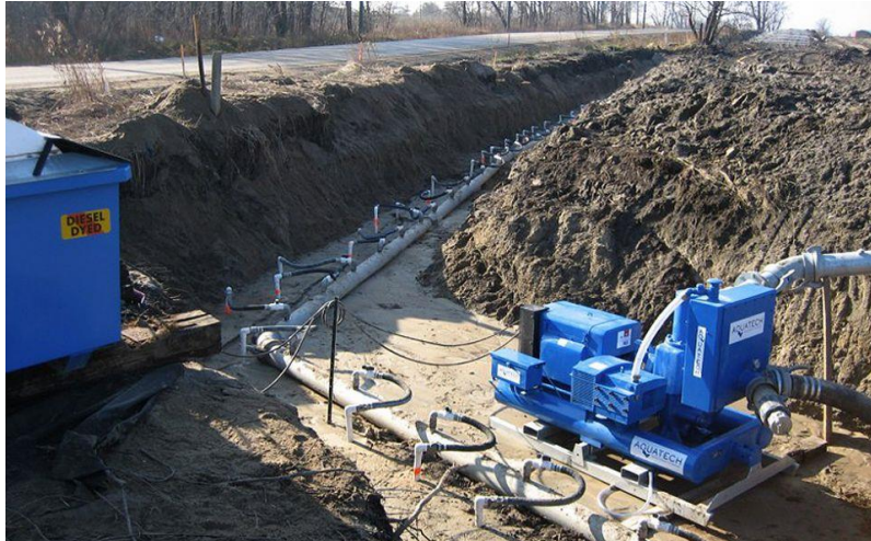
Figure 4.12.1 Dewatering using well point system on site (from google website)
