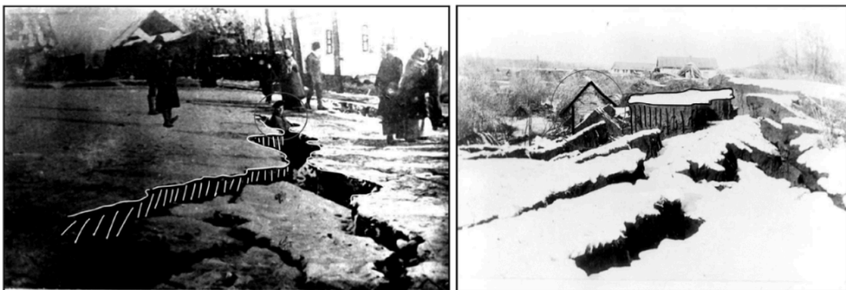
Figure 2.3. Almaty's ground failure (Kemin earthquake)
