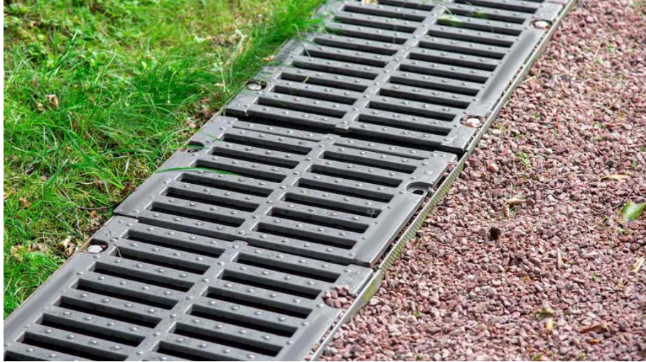
Figure 80. Trench open channel example
