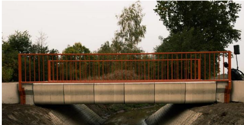
Figure 9. Gemert's 3D-printed bicycle bridge [58]
