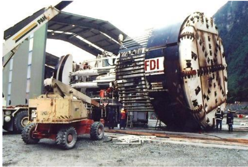
Figure 3.2. TBM utilized for the Manapouri Second Tail Hydropower Tunnel (Kim, 2004)
