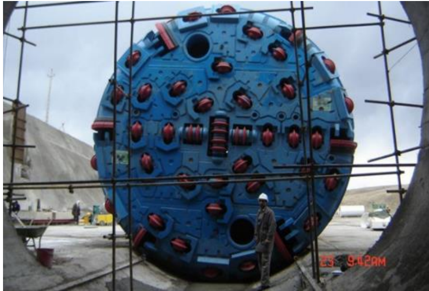
Figure 3.6. TBM utilized for Zagros Water Transfer Tunnel (Goodarzi, et al. 2021)
