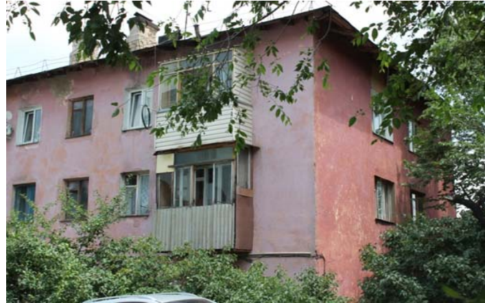
Fig: 4 Unreinforced Masonry with adobe bricks
