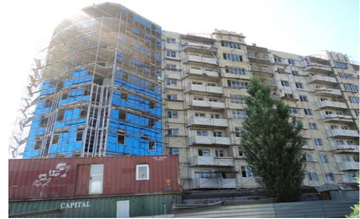
Fig: 6 Reinforced Concrete
