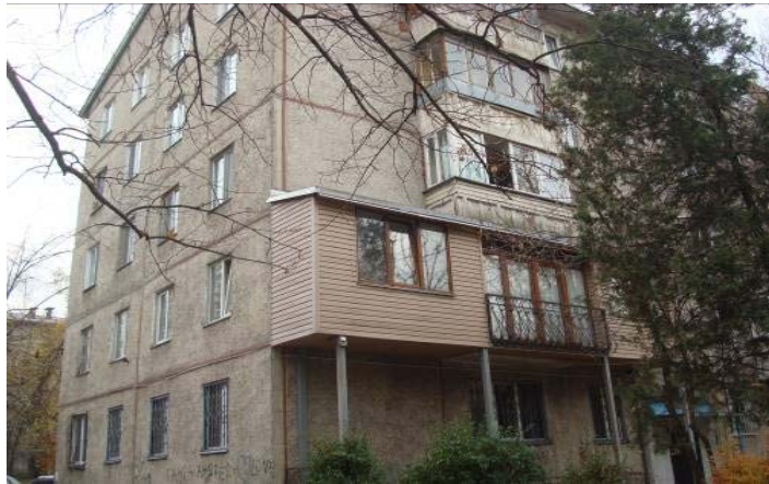
Fig: 5 Pre-cast Concrete Wall Panels
