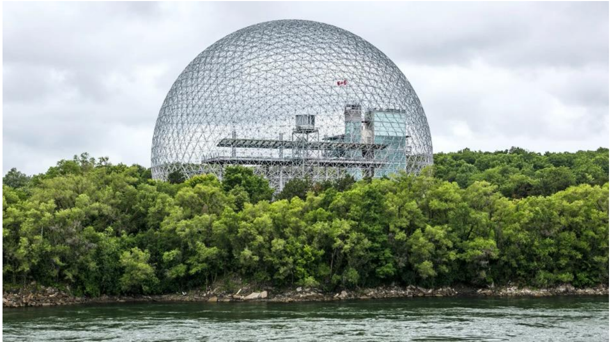
Figure 34: Famous geodesic dome project for the Expo 1967 in Montreal, Canada by Buckminster Fuller
