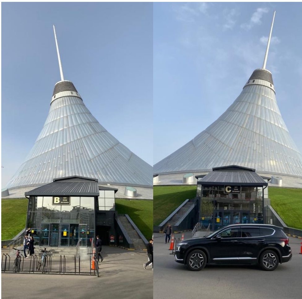
Figure 54: Additional pedestrian entrances to Khan Shatyr. Photo by the author
