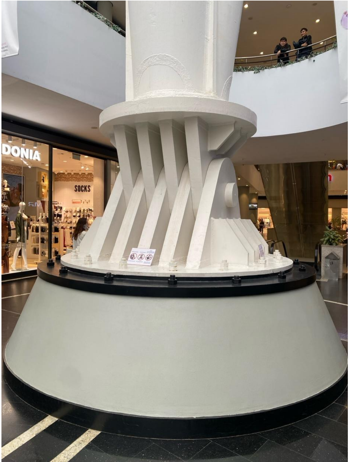
Figure 40: The moving leg of a tripod which was the main leg when it was mounted into place by hydraulic cranes. Photo by the author 2025
