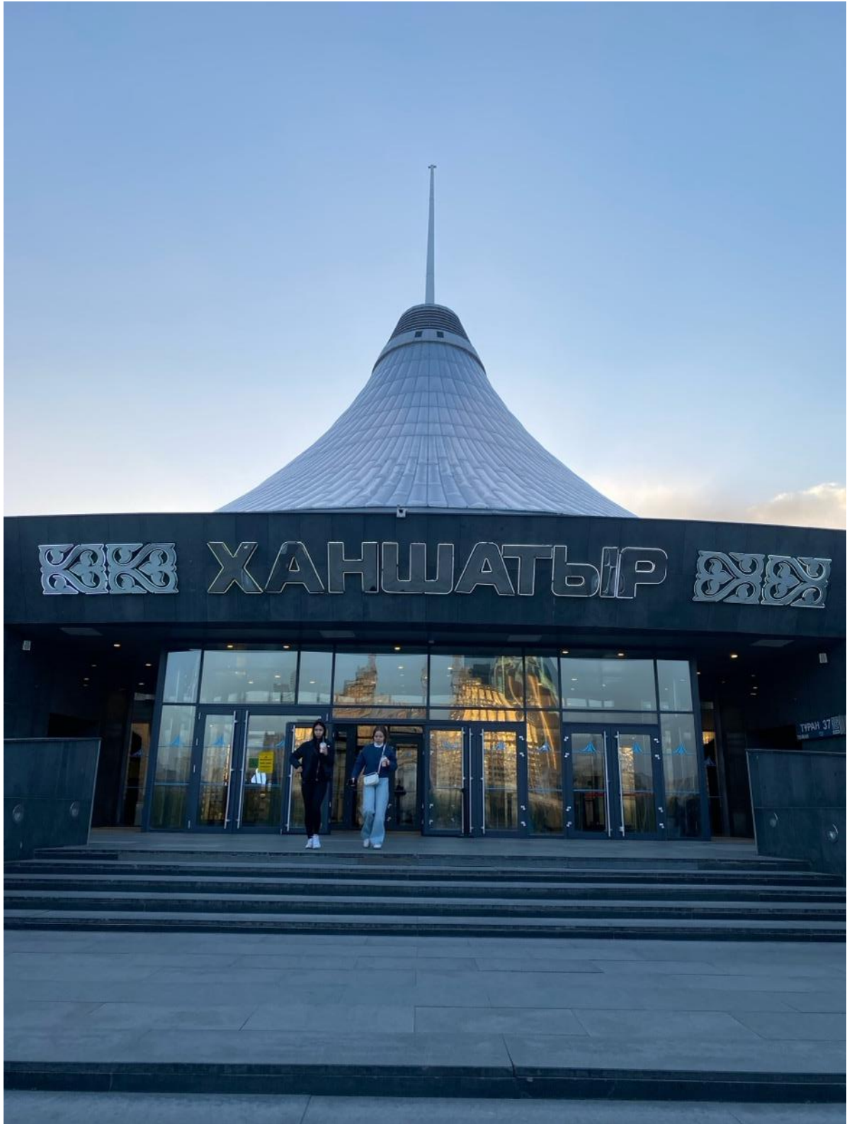
Figure 29: Khan Shatyr main entrance which is located on the west end of the Nurly Zhol Boulevard. Photo by the author 2025
