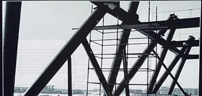
Figure 9: Construction process. The uplifting the “Cradle of the world” made of steel structure prefabricated in Britain and assembled on site in Astana. Photo by the author 2025
