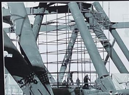
Figure 9: Construction process. The uplifting the “Cradle of the world” made of steel structure prefabricated in Britain and assembled on site in Astana. Photo by the author 2025
