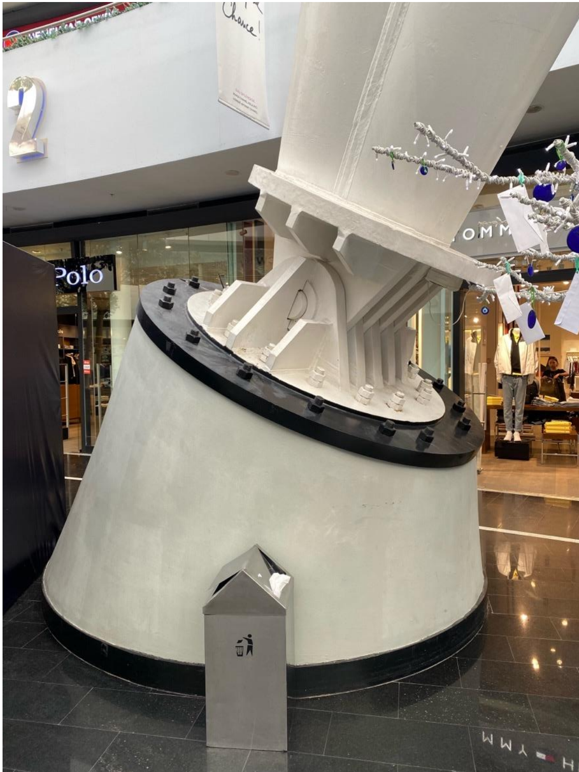
Figure 39: One of the legs of a tripod that is firmly fixed to the concrete foundation by steel nuts and bolts. Photo by the author 2025
