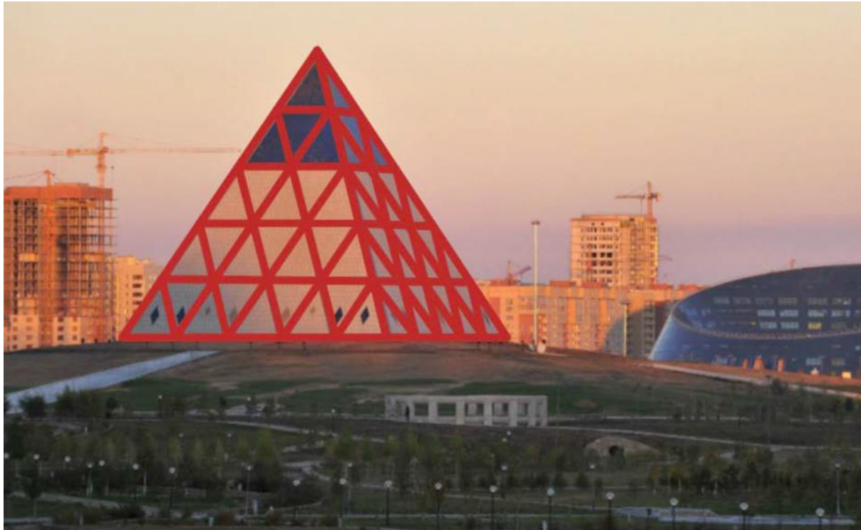
Figure 23: The main structure of the Pyramid is a diagrid which is a structural system composed of diagonally intersecting metal, concrete, or wooden beams. Diagrids reduce steel usage, improve load distribution, and increase design flexibility. Structural analysis
