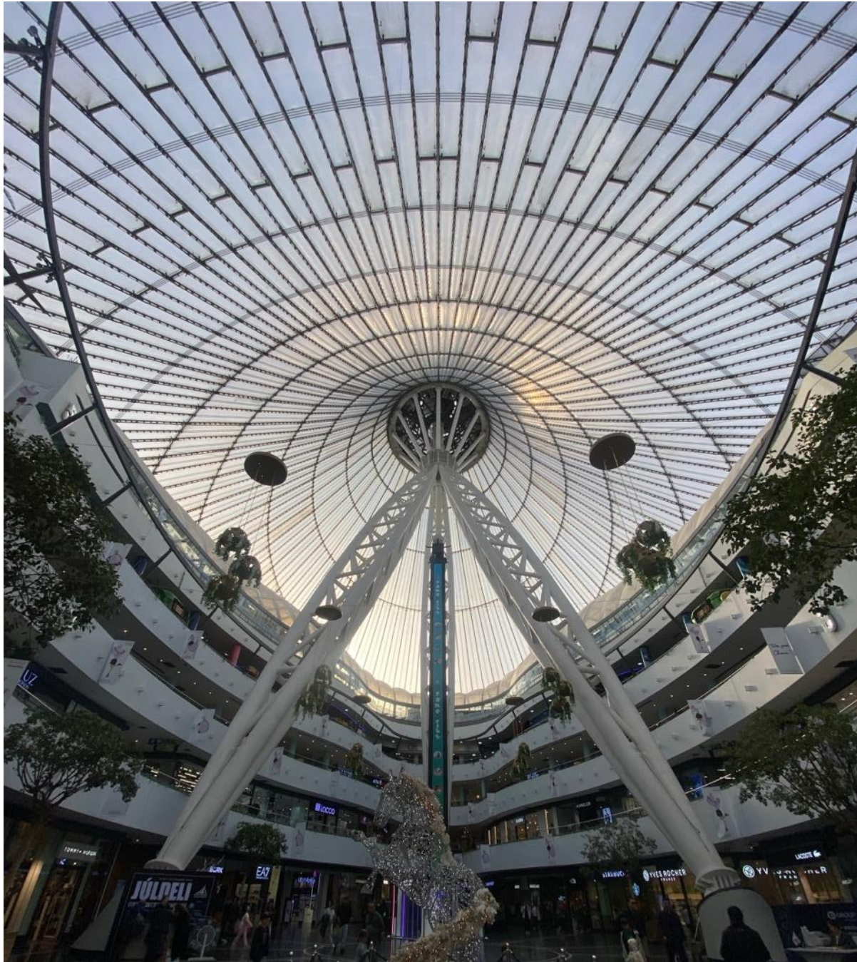
Figure 38: Amazing view inside of the biggest tent in the world. Steel tripod holding the weight of an entire metal cable and ETFE. Photo by the author 2025
