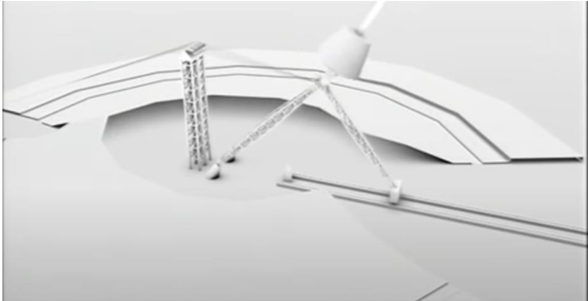
Figure 44: Khan Shatyr computer model that help visualizing the lifting of a steel tripod. Online documentary
