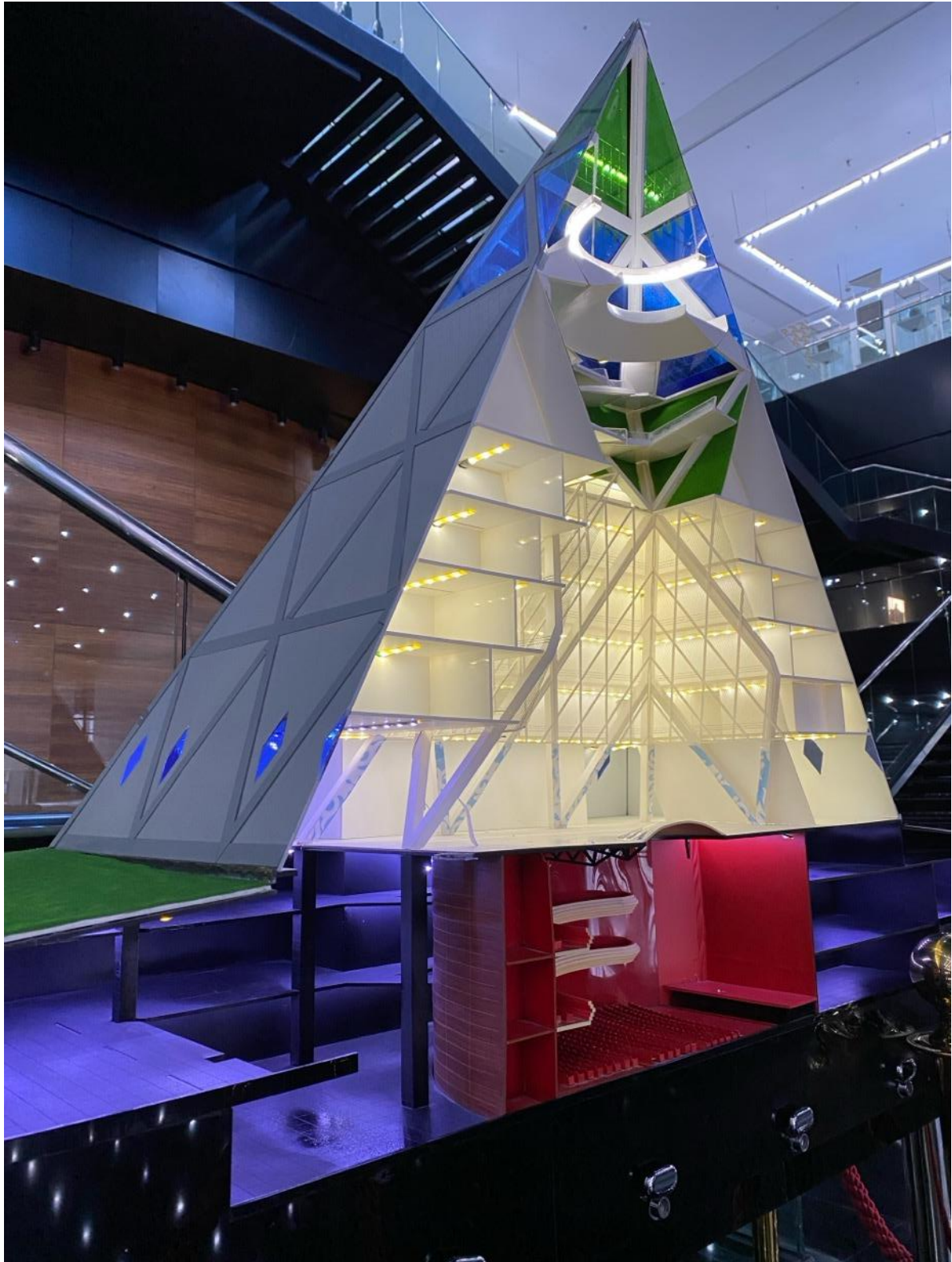
Figure 22: Physical model of the Pyramid, side section that shows the interior working of the building. Structure, levels and vertical circulation. Dark underground level with red opera hall in the middle. Photo by the author 2025
