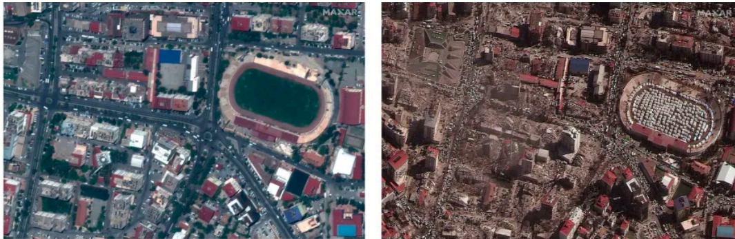
Figure 11. The satellite images taken before and after the earthquake (Maxar Technologies)
