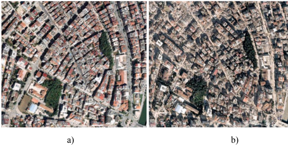
Figure 13. Satellite imagery of a) pre-earthquake and b) post-earthquake for Antakya
