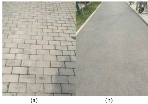
FIGURE 5. a) Block road, b) Asphalt road.
