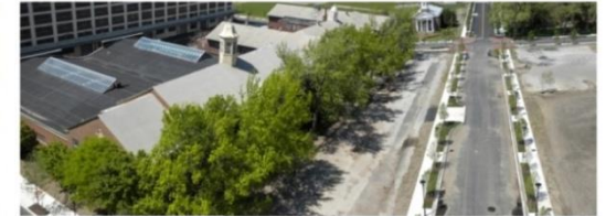
ROOF & PARKING LOT
