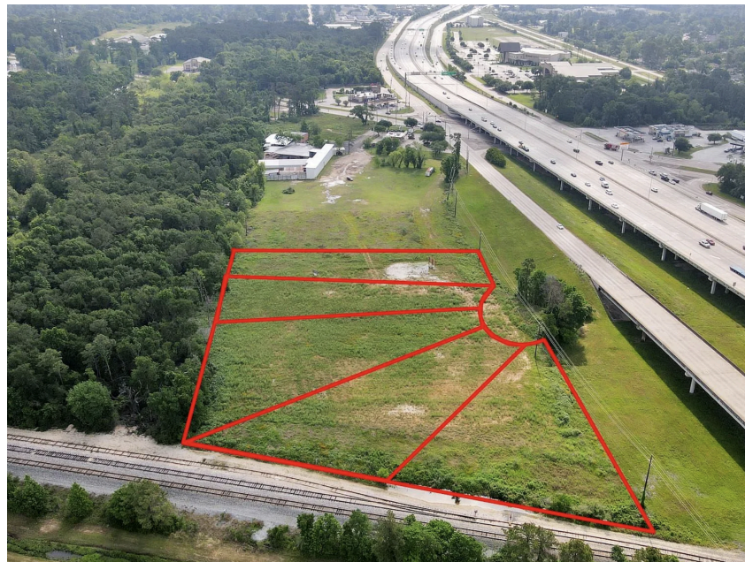
Figure 6.2.2 3D view of the construction site
