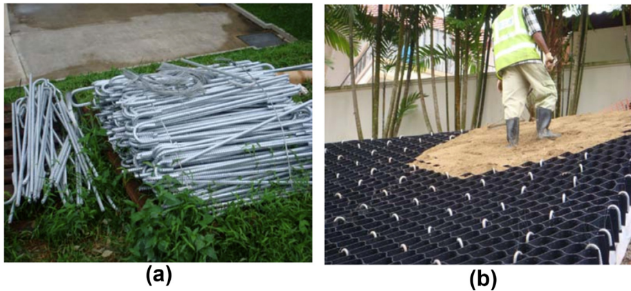
Fig. 4. J-pins before (a) and after (b) installation.
