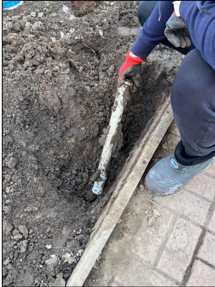
DEV-4. Placing PVC pipe under the ground.
