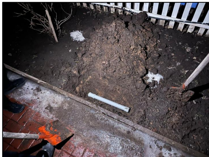
DEV-5. Buried setup inside of the isolation tube.
