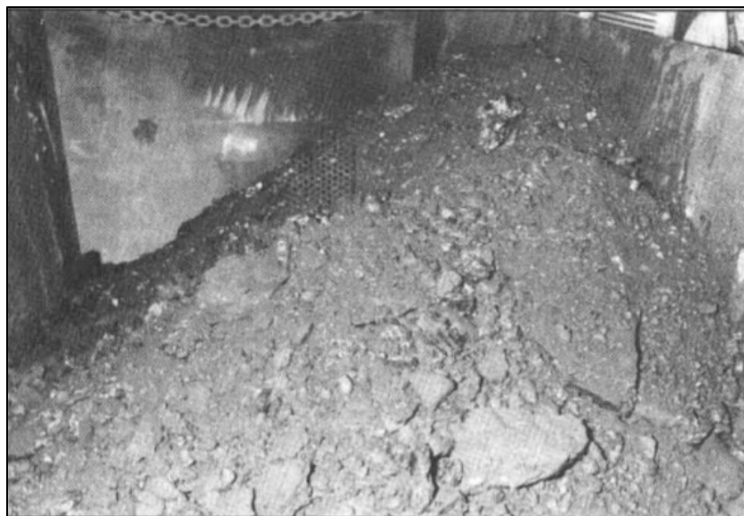
Figure 18 - Asphaltene debris that was removed from the separator [47].
