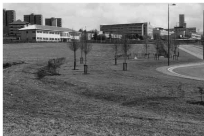
Figure 2. Conveyance swale (Woods-Ballard et al., 2007)
