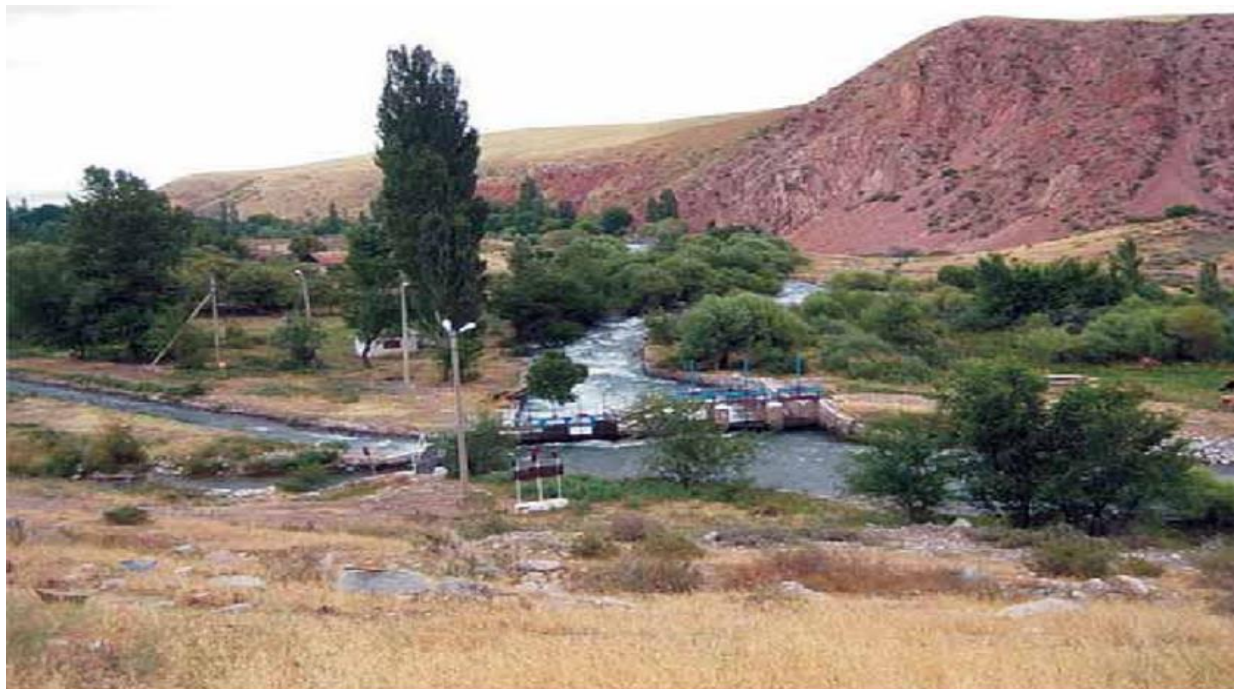
Figure 3. Water distribution unit on Aspara River Source: USAID, 2015.
