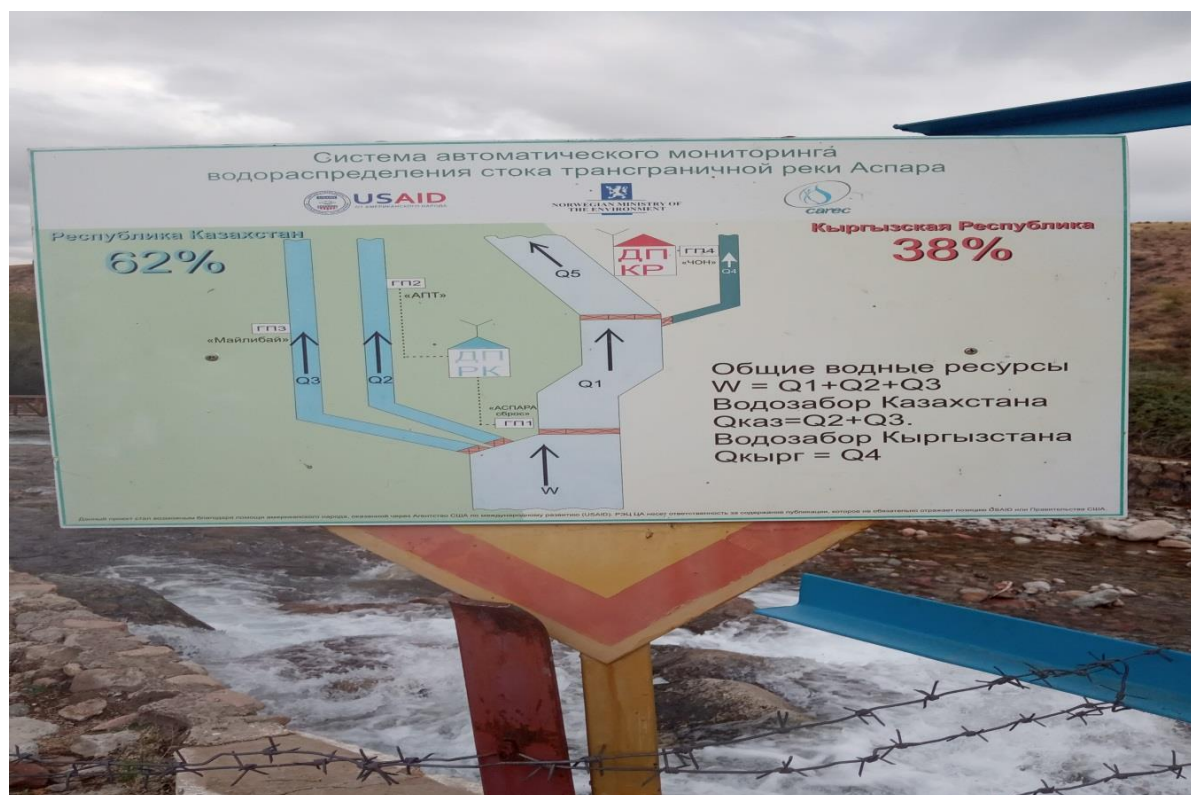
Figure 4. Scheme of runoff water allocation automatic monitoring system of the Aspara River. Source: USAID, 2015
