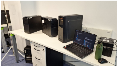
Fig. 1. One of the servers running the project backend
