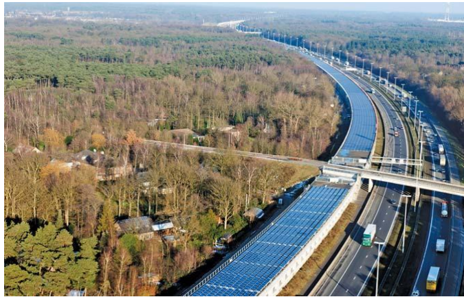
Figure 2. 2: The first solar-powered railway tunnel in Belgium, taken from [17]
