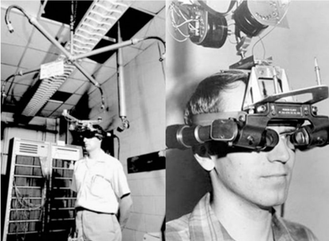
Figure 2.1: Sword of Damocles, one of the early systems for AR by Ivan E. Sutherland.
