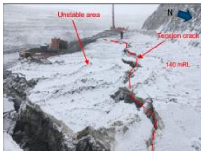
Figure 1.1: An example of tension crack during field inspection.
