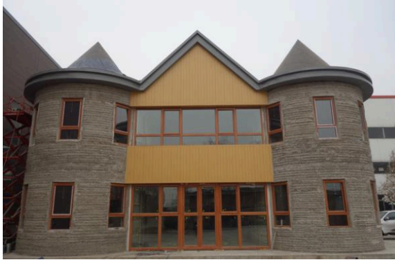
Figure 5. 3D printed house by HuaShang Tengda
