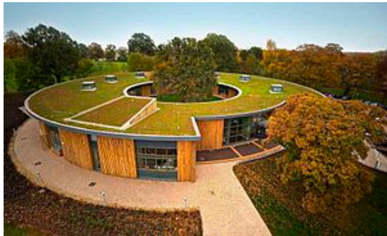
(a) Extensive green roof
