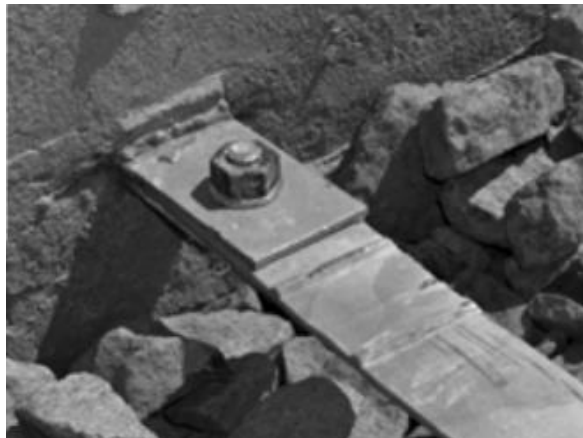
Figure 5. 7 Panel to strip bolted connection
